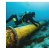
SUBSEA CABLE INSTALLATION
